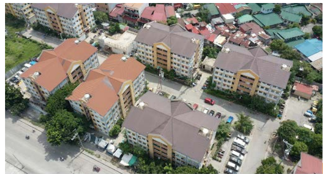
The second phase of the APOAMF-LRBP has been completed, with six buildings housing 360 families.
