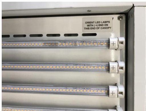
Figure 6-1 LED Tube Orientation
