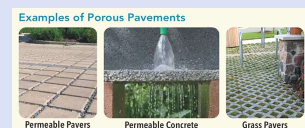
Fig 7: Different types of porous pavements [8].
