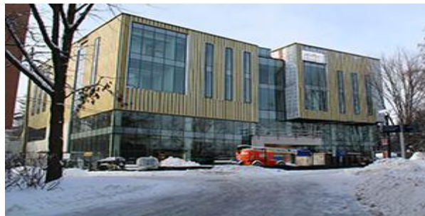
North Building Reconstruction – “Deerfield Hall” Photo by Gareth
