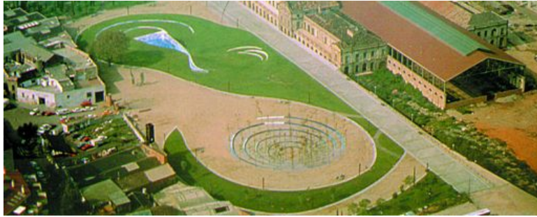
Precedent - UTM Quad Informal Amphitheatre created with level change Parc de l'Estacio del Nord, Barcelona by Cubiertas y Mzov
