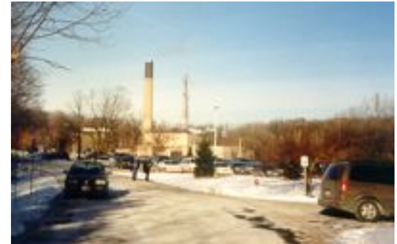
UTM - Main Utility Plant
