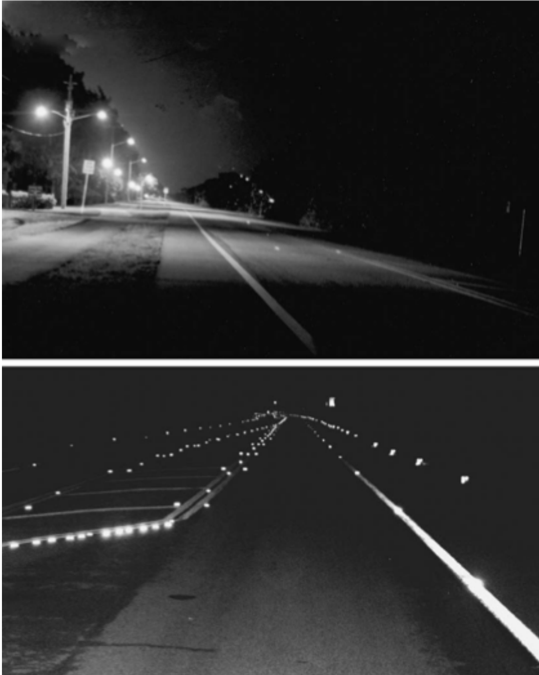
Figure 5. A comparison between unshielded streetlamps (top) and embedded road lights (bottom) from Bertolotti and Salmon (2005). Unshielded streetlamps cast a high amount of unnecessary light around a greater surface area. In addition, they also cast upwards light and contribute to sky glow. On the other hand, embedded road lights are low to the ground and cast enough light to dimly light areas where needed (Bertolotti and Salmon 2005).
